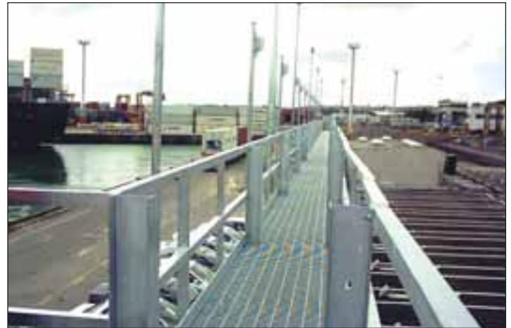
Container Loading Dock
