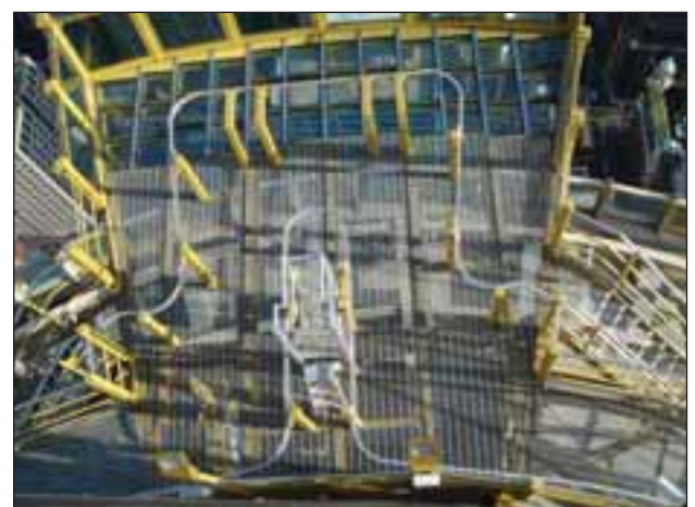
Platform Top View
