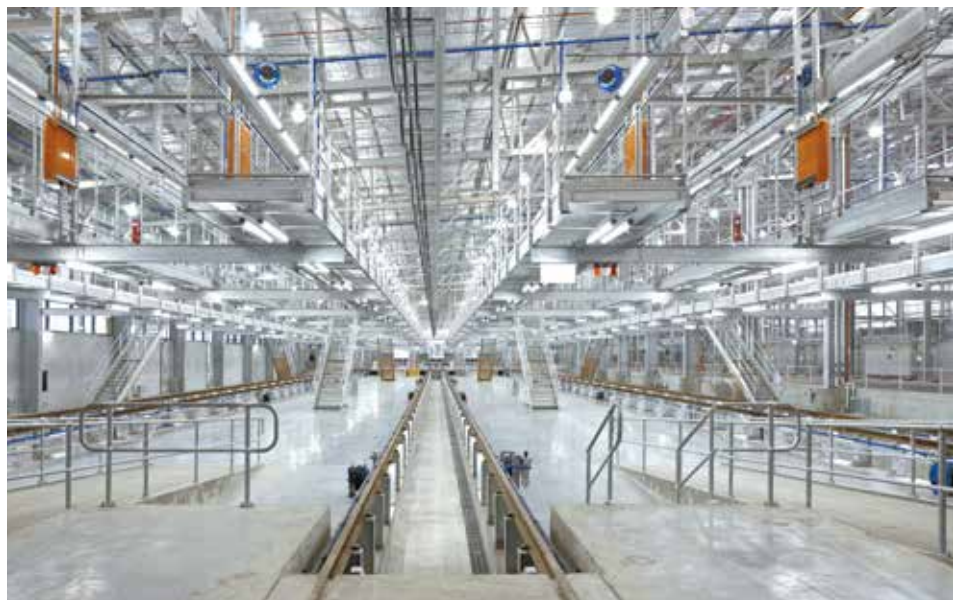
Inside of Craigieburn Train Maintenance Facility
